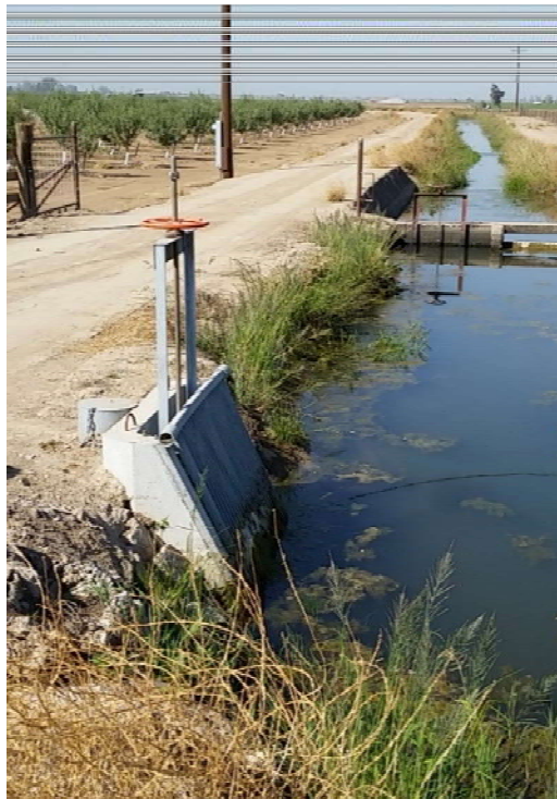
Figure 6-5 Canal Turnout Gate with Trash Rack
