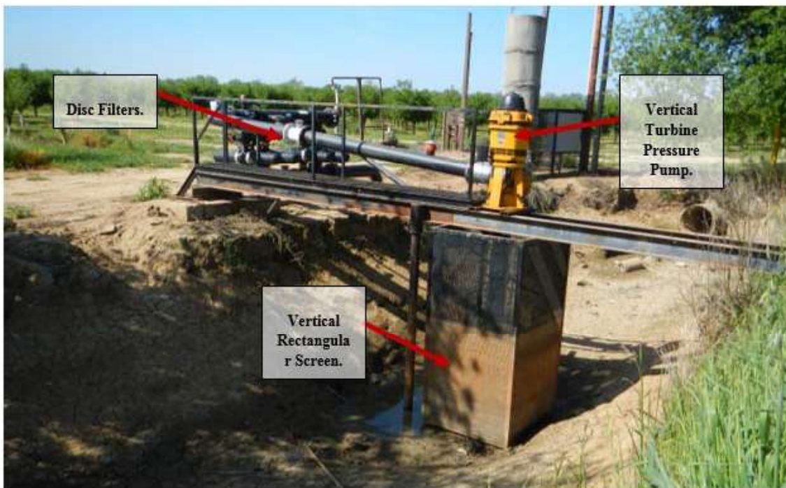
Figure 6-11 Vertical Rectangular Screen Protecting Vertical Turbine Pressure Pump, Followed by Disc Filters for Prune Irrigation with Microspray
