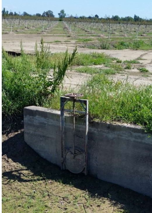
Figure 6-5 Canal Turnout Gate with Trash Rack
